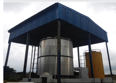
Image source: Biogas plant at VFSTR
